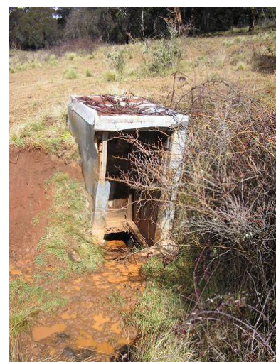
Figure 2 Air vent to Bi Mine
