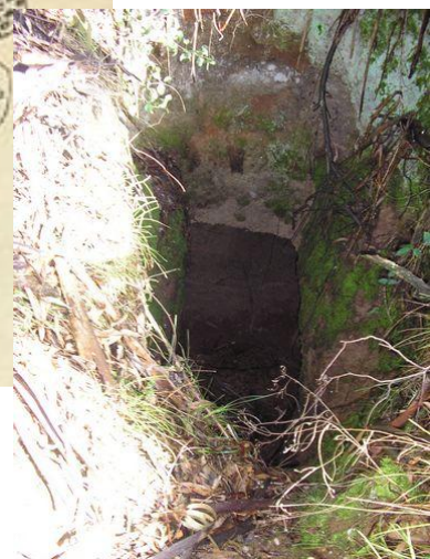
Figure 3 Ventilation Shaft at NW End of area
